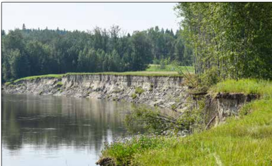
Massive erosion visible off a field on Township Rd 593A.
