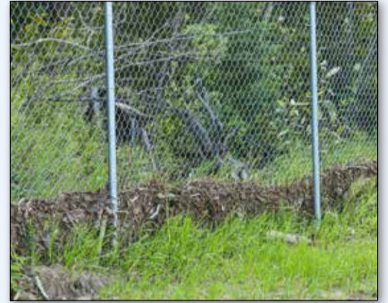
Muddy debris along the fence line.
