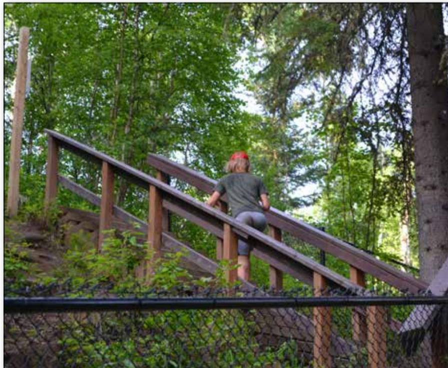
A portion of the stairs at Hard Luck Canyon.
