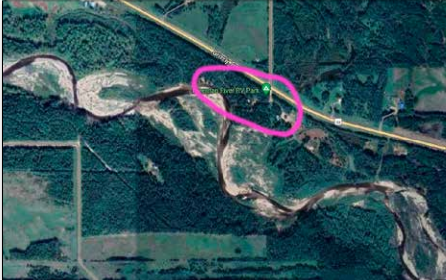
The Freeman River RV Camp (circled) in-between Hwy 33 (above) and winding river (below).
