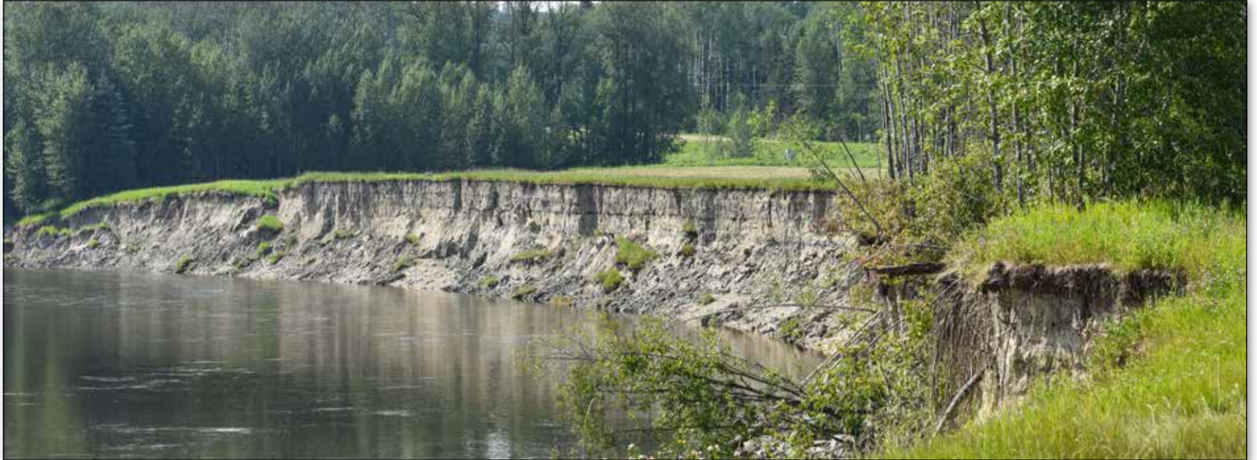
The very eroded riverbank near the intersection of Old Ferry Road and RR 1245.
