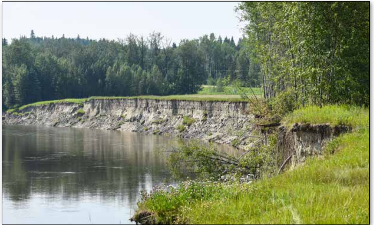
One vantage of the eroded river bank on Old Ferry Road.
