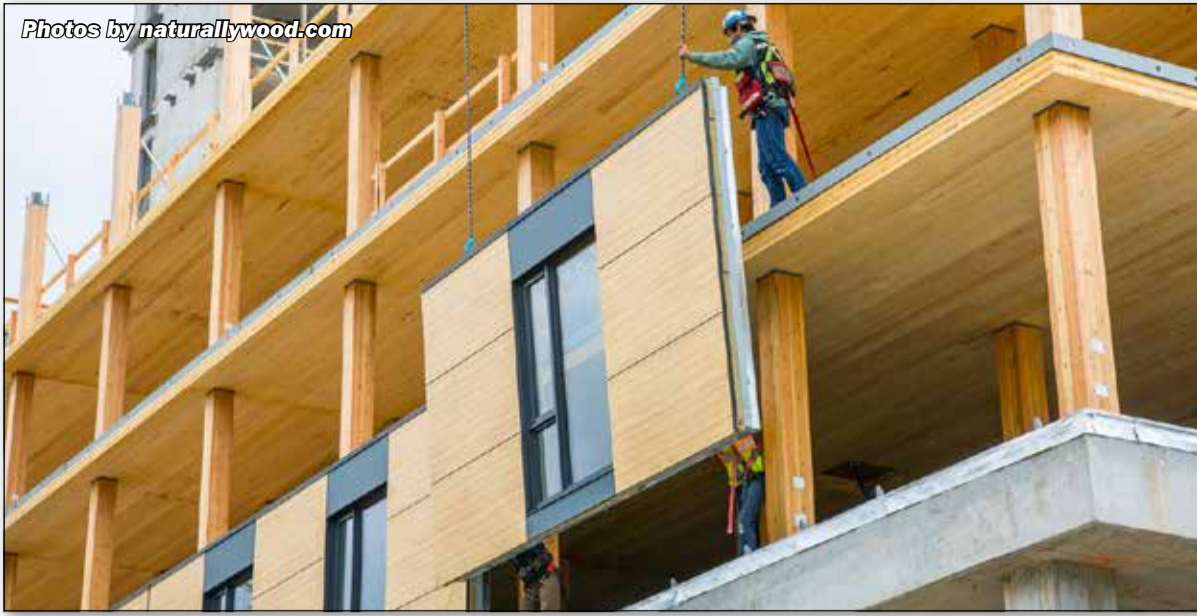
Prefabricated pieces resulted in a speedy rise for the 'Woodscrapper'.
