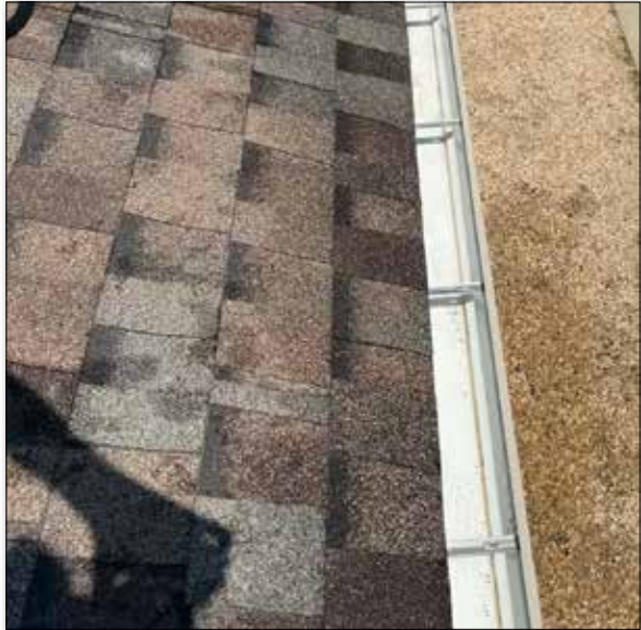
Before and after: Cleaning out eavestroughs is one of the fall maintenance jobs that can help prepare a home for the winter months. Removing leaves and debris allows water to drain properly and helps prevent potential problems when snow and ice arrive.
